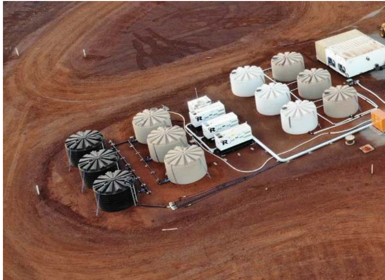
Figure 10. Potable Water Holding Tanks
