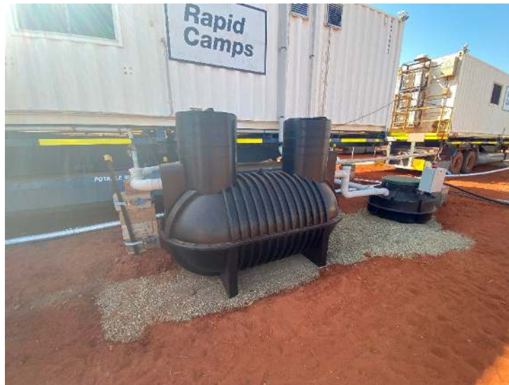
Figure 15 Grease Trap
