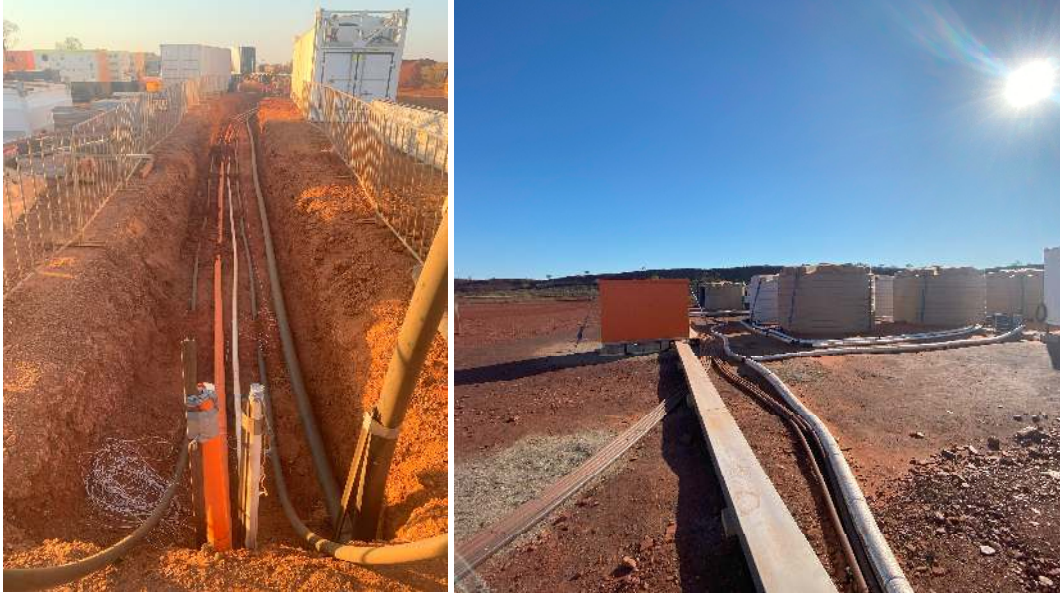
Figure 11 In and above ground potable water and power
