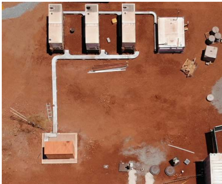
Figure 2. Generators and Fuel Pod Configuration
