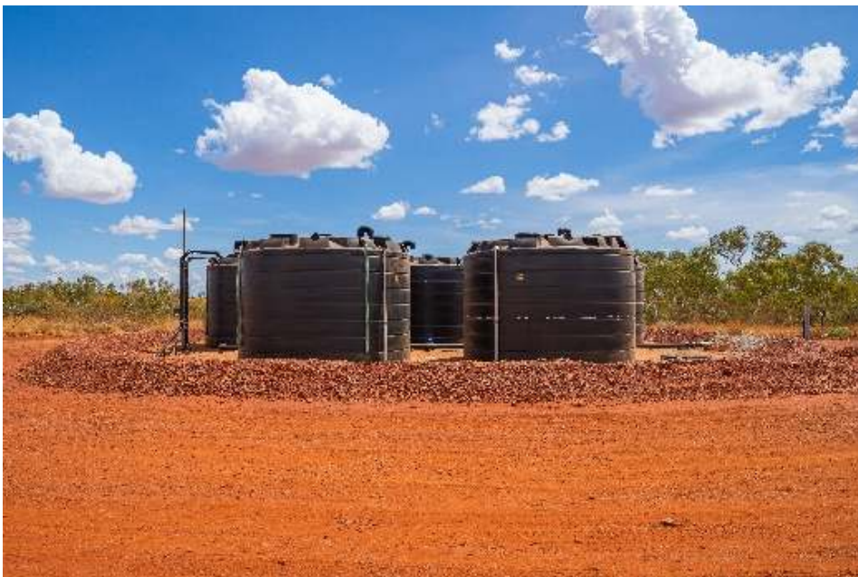
Figure 13. Waste Water Holding Tanks
