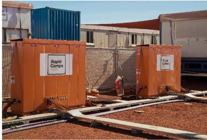
Figure 6. Site Main Distribution Boards
