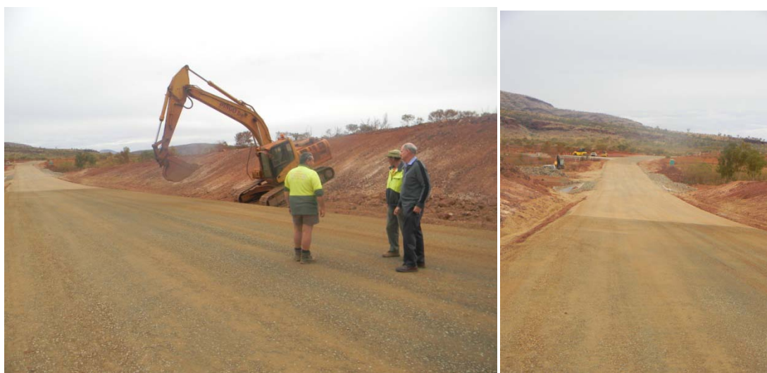
Roadworks – Nanutarra-Munjina Road
