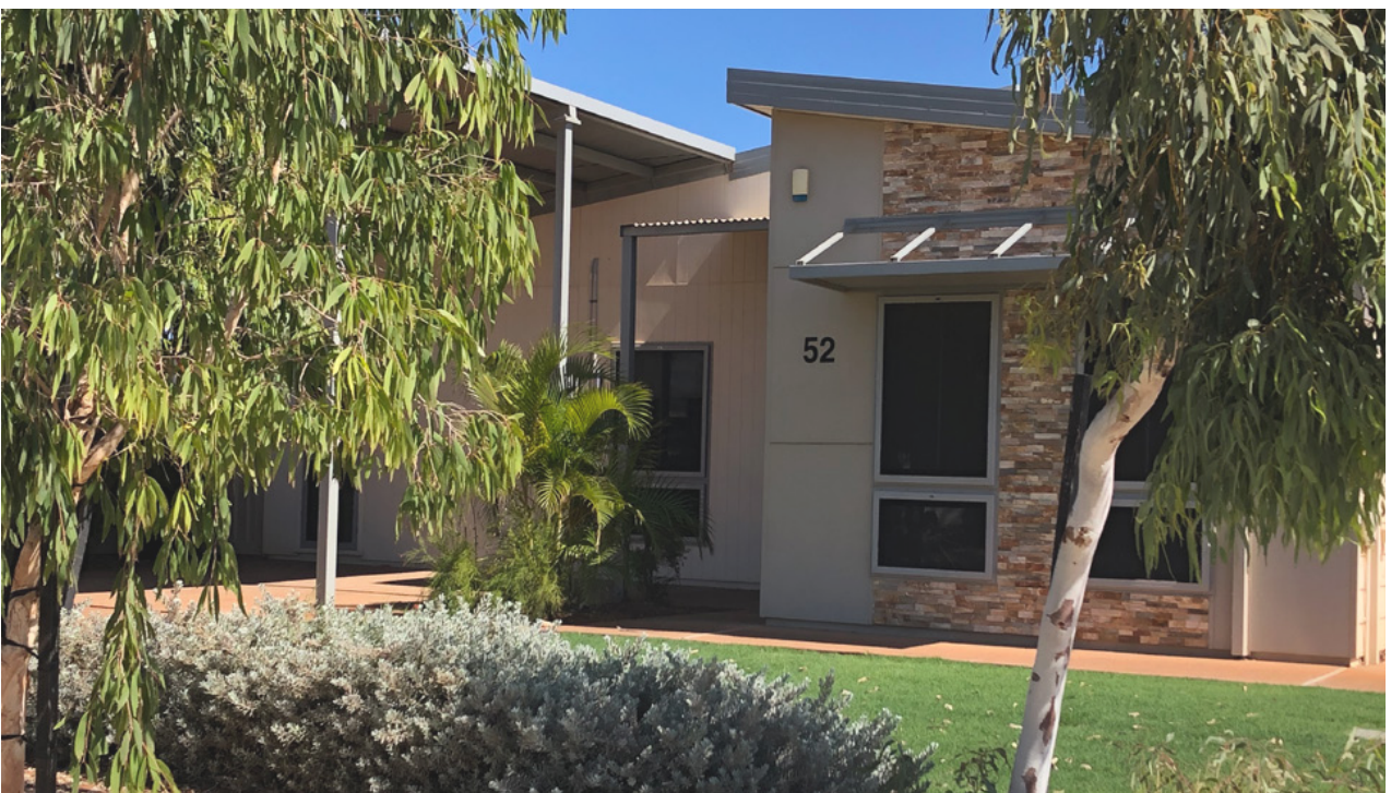
6 Carlyon, Onslow - New Build
