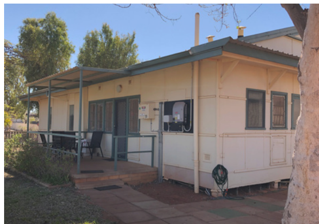
Transit House, Onslow
