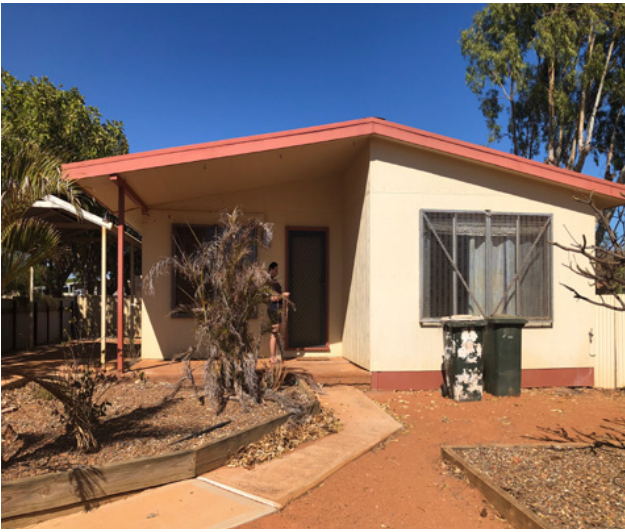
583 Third Ave Onslow (Proposed Demolition)
