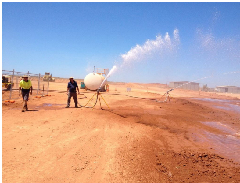
Figure 3.9: Sprinklers set up near the turkeys nest to pre-condition the select fill
