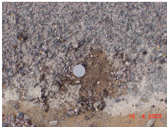
Figure 2.6: Salt damage on shoulder widening constructed with full depth sea water, 5 months old
