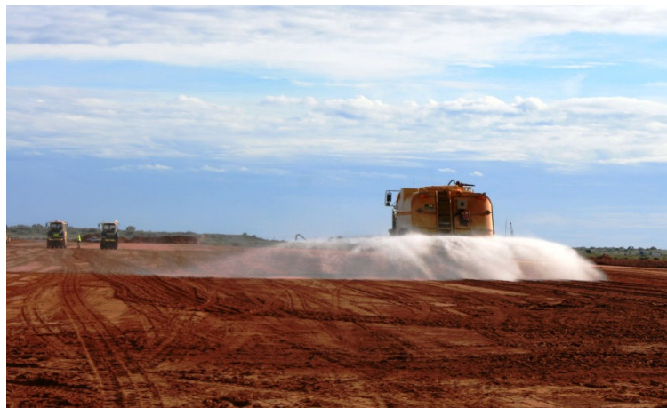
Figure 3.7: Sea water applied to formation works
