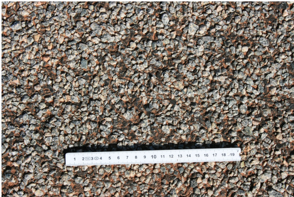
Figure 3.11: Sprayed seal on existing runway
