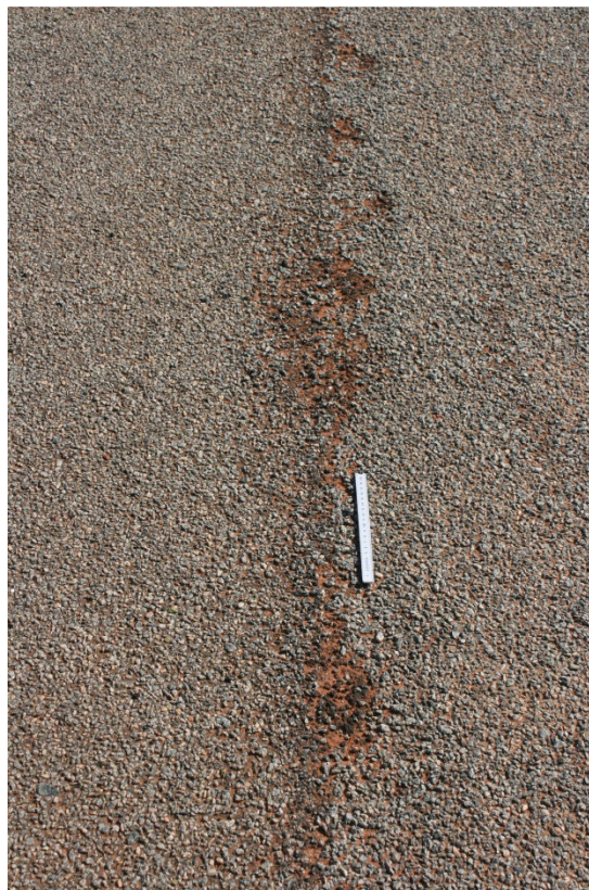
Figure 3.15: Salt damage
