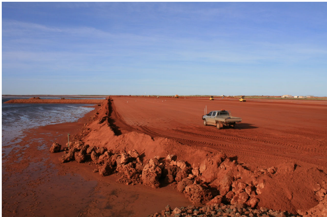
Figure 3.3: Proximity of sea water to the runway earthworks
