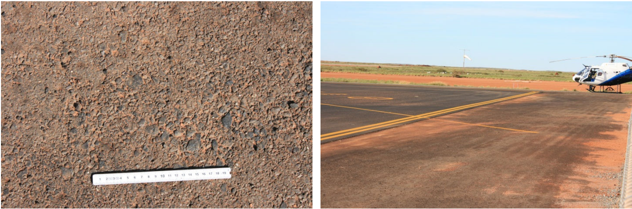
Figure 3.19: Site trial of basecourse material compacted with sea water, primed and asphalted
