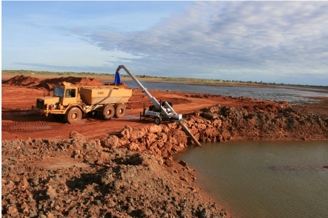
Figure 3.6: Sea water for compaction is extracted from adjacent to the earthworks
