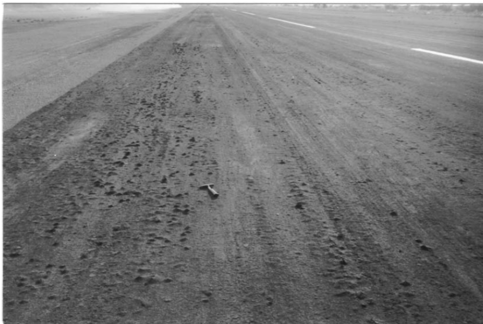
Figure 2.7: Volcano blisters and salt in loosened primed base
