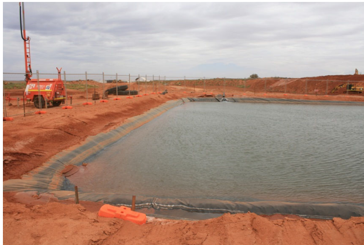
Figure 3.8: Seawater stored at the 'turkeys nest'
