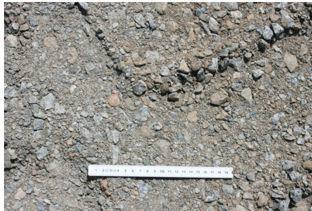
Figure 3.17: Basecourse material (compacted under the tyre of a front end loader)
