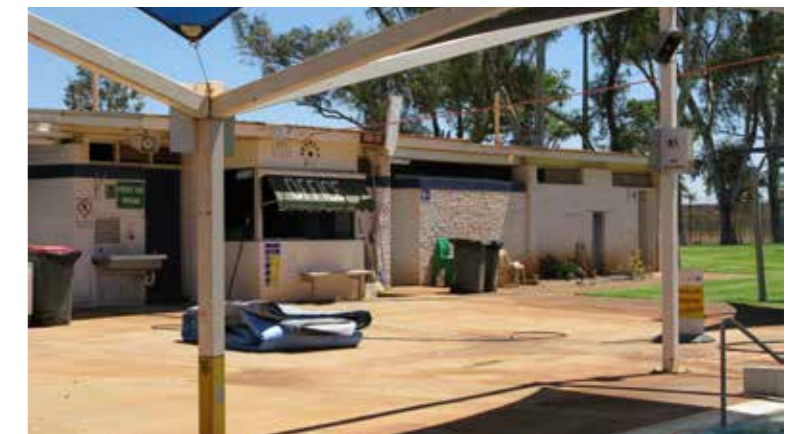
Swimming pool change rooms and office building to be demolished
