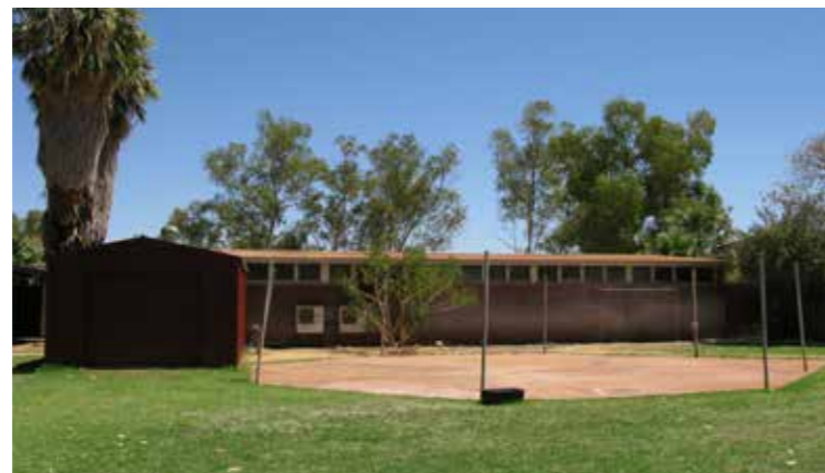
Paraburdoo library view from Community Hall courtyard
