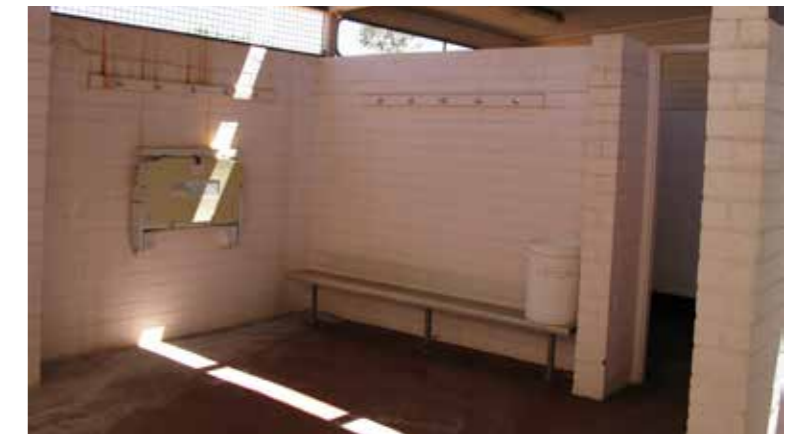
Swimming pool change rooms to be demolished
