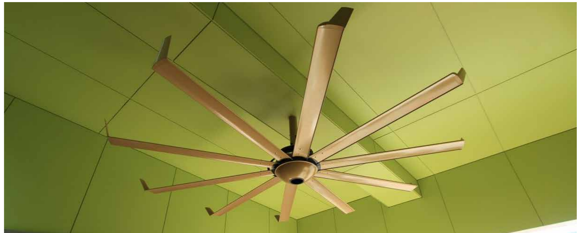
High Volume Low Speed (HVLS) fan to assist with external and internal thermal comfort.
