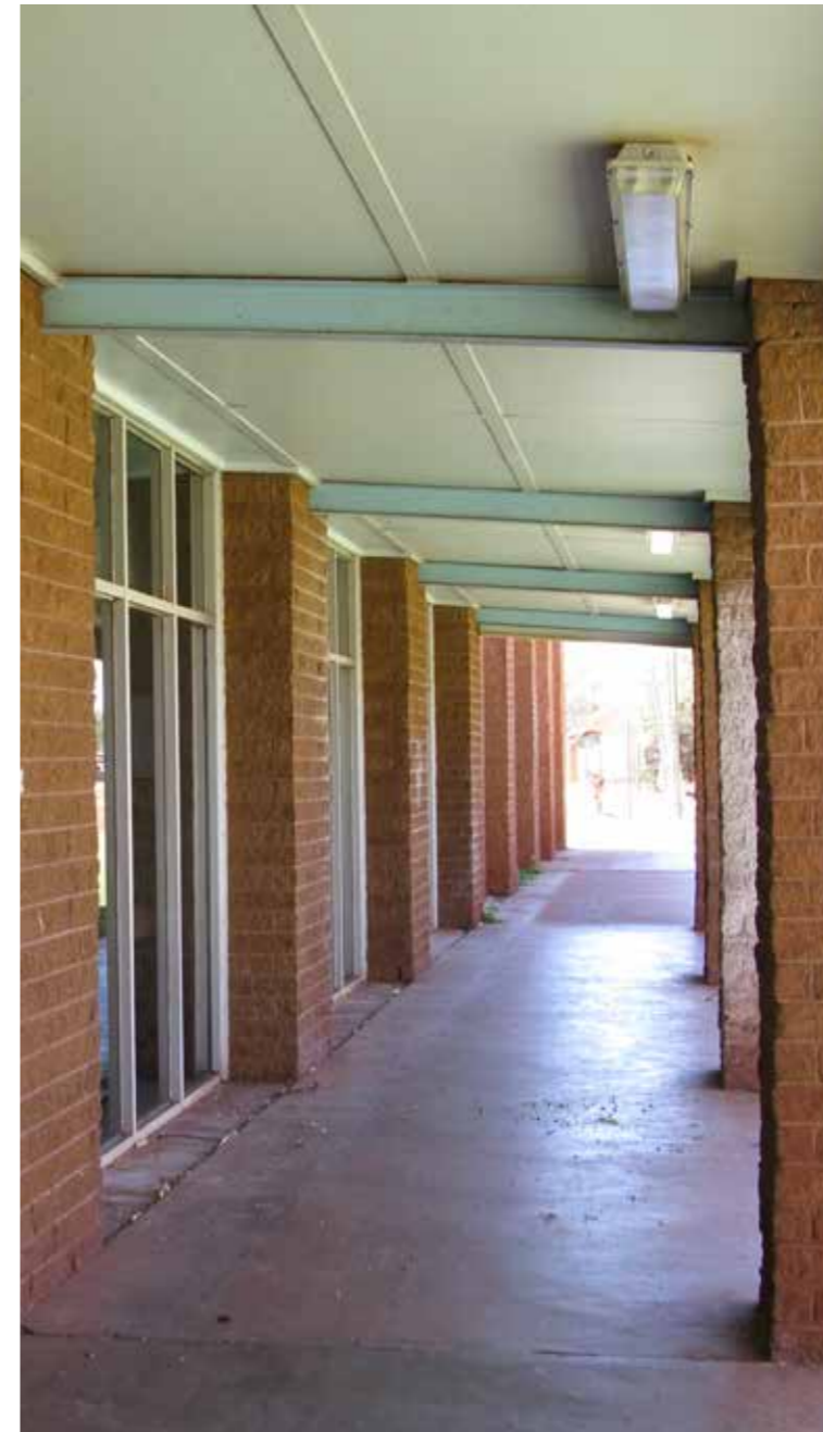
Sports pavilion perimeter verandah
