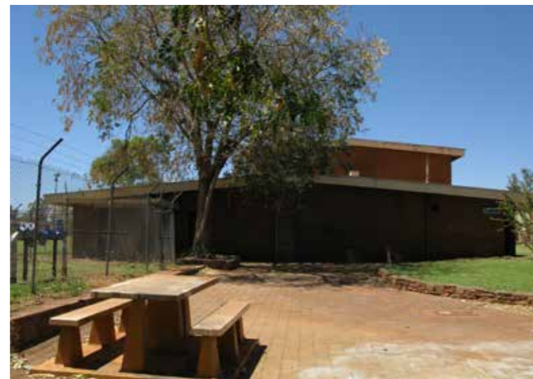
Outdoor area adjacent to sports pavilion, west facade
