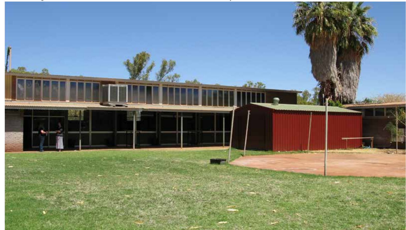
Community Hall courtyard and red storage shed
