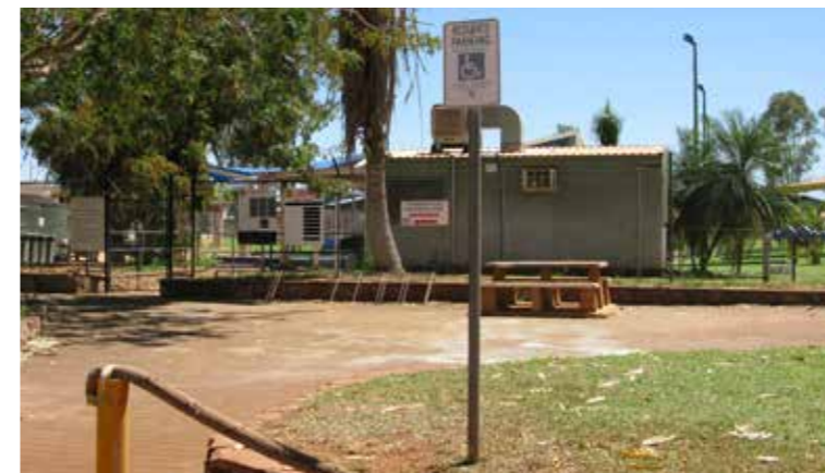
Kiosk adjacent to swimming pool to be demolished
