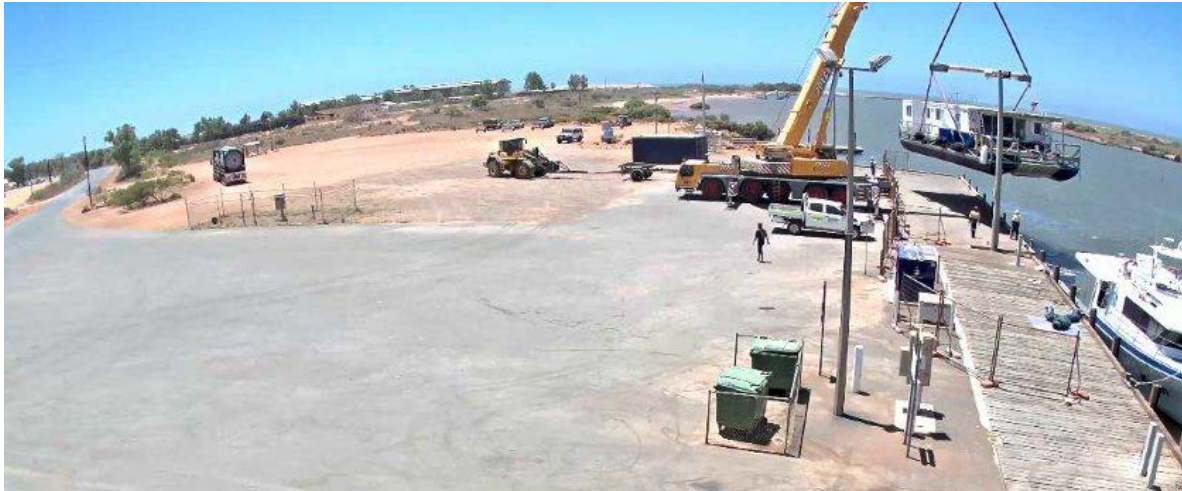
Figure 1 Larger Vessels Require Lift
