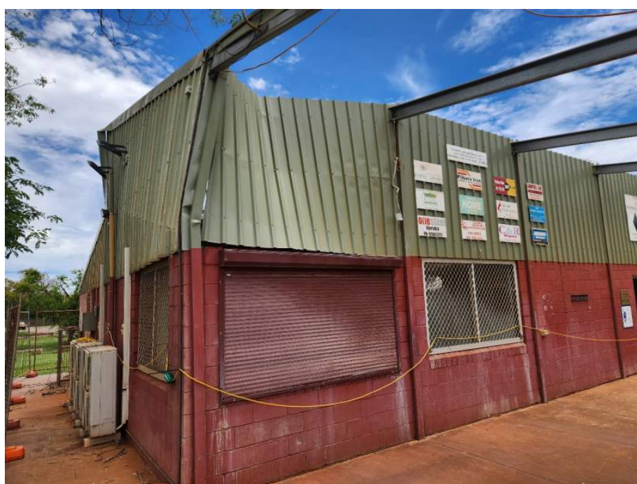
Photo 6 - General view of the observed damage to the patio roof and wall cladding
