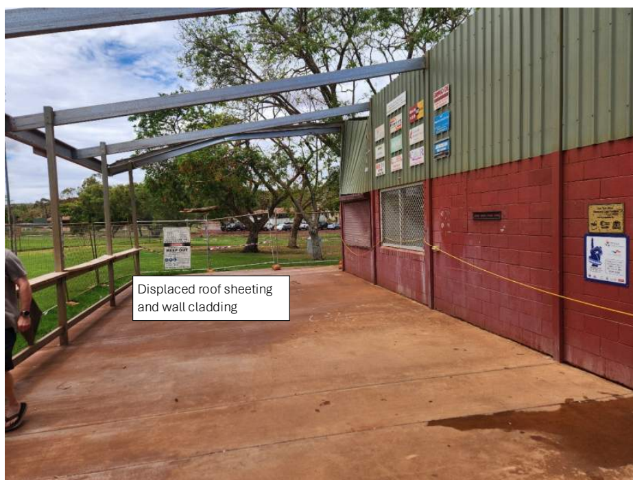
Photo 5 - General view of the observed damage to the patio roof
