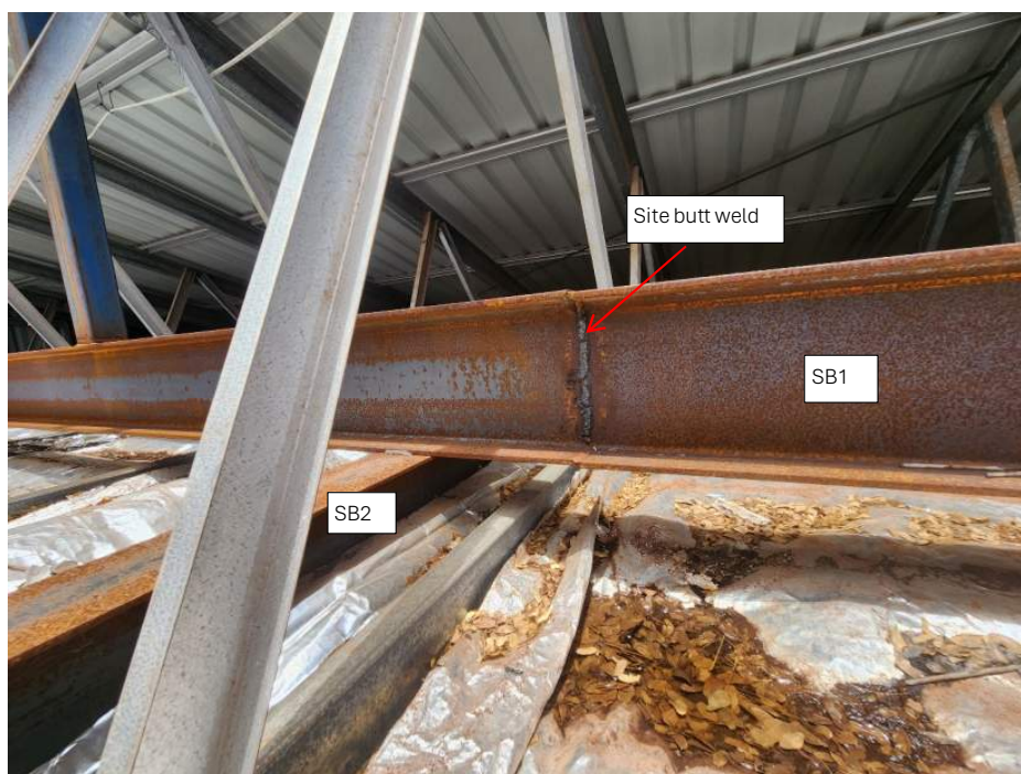
Photo 15 - General view of connection between strutting beams – refer enclosed drawing
