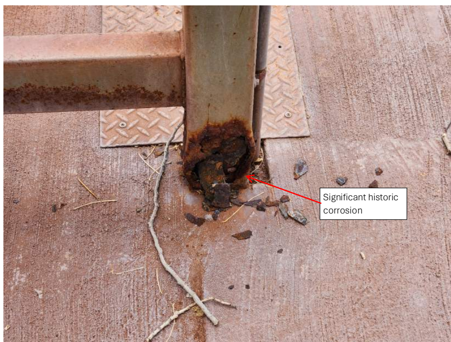
Photo 7 – Example of observed corrosion damage at base of veranda post
