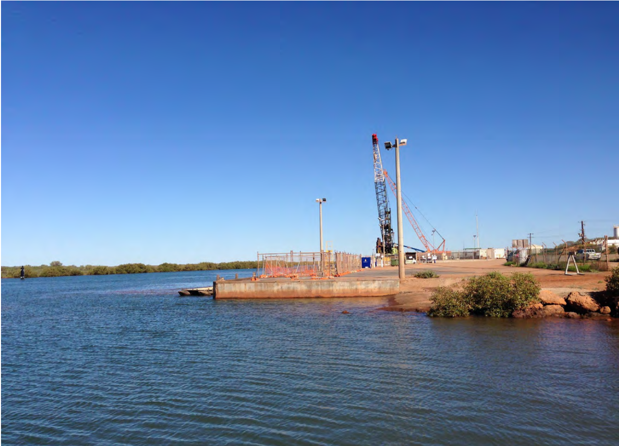
12.12 - 2023/24 - Construction site near the water's edge.
