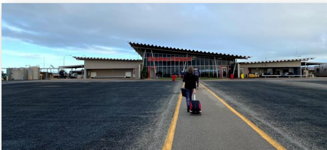
Figure: Onslow Airport
