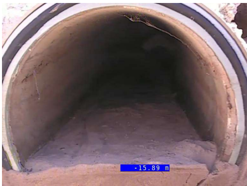
Chainage: ? - STMH - Start node - Maintenance hole
