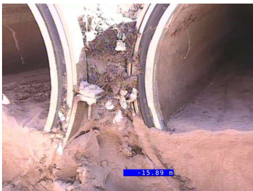
Chainage: ? - STMH - Start node - Maintenance hole
