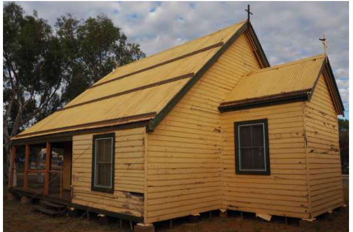
Side and rear elevations of church, 2016.
