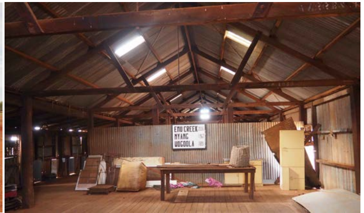
Inside view of Shearing Shed, 2016.
