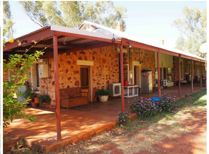
Hamersley Homestead rear elevation, 2016.
