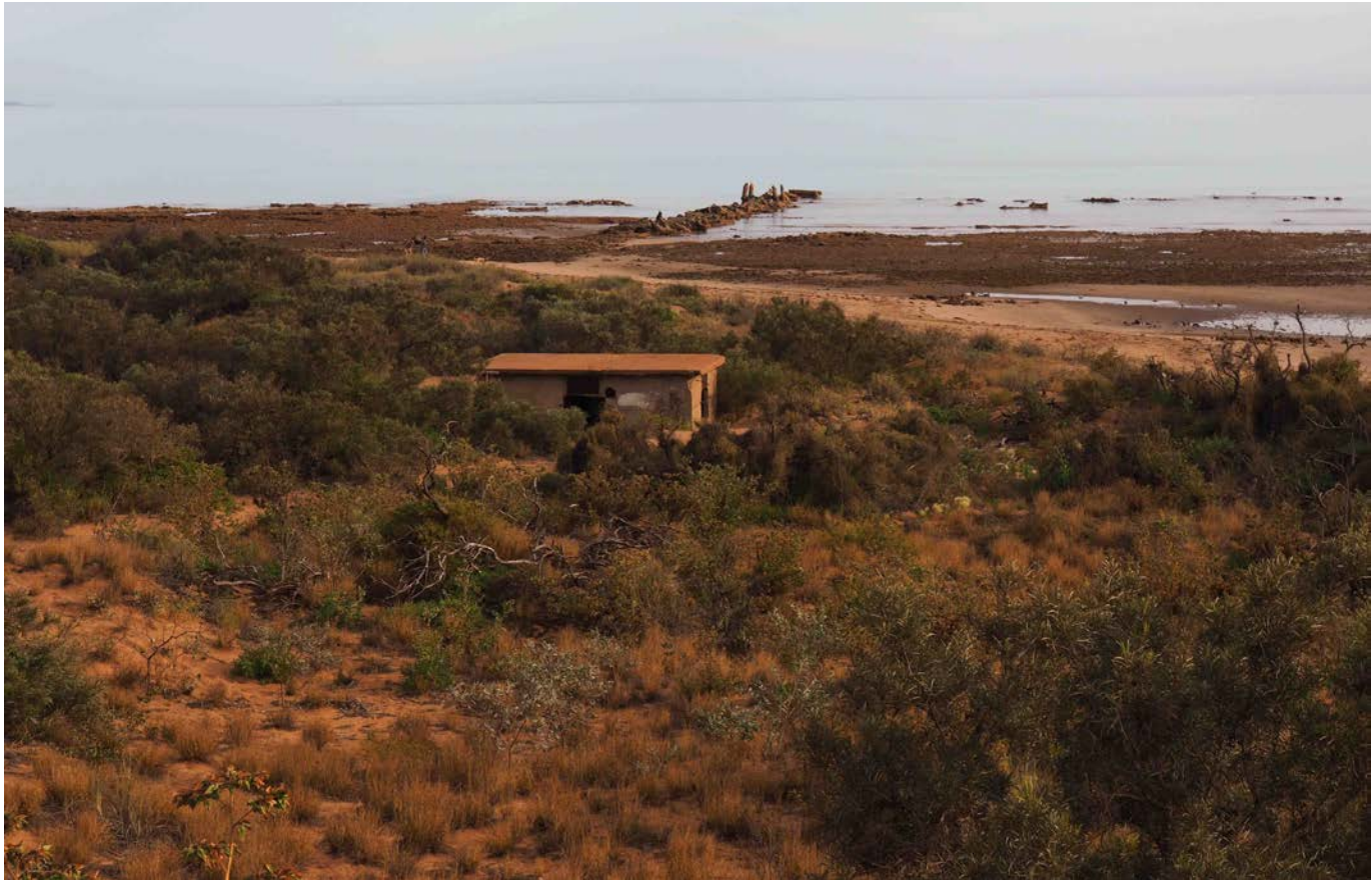
Pump Out Station and remains of Onslow jetty beyond, 2016.
