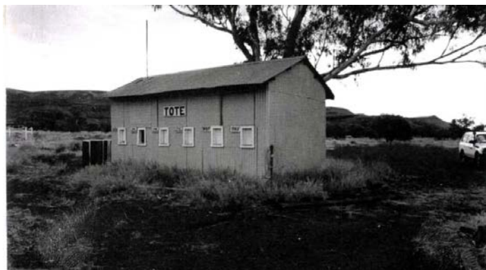
Left image: Wittenoom Racecourse, 1995 (demolished 1995). Source: National Trust of Western Australia (1995)
