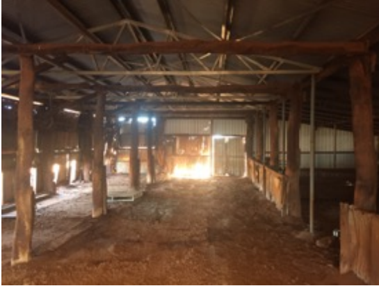
Inside Shearers Shed with bush pole structure, 2017
