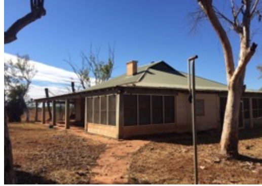
Homestead infilled verandah, 2017
