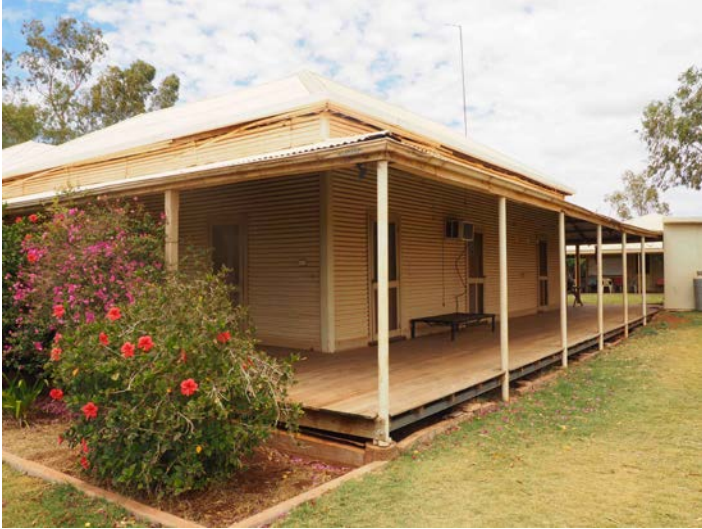
Western elevation of Yanrey Homestead, 2016.
