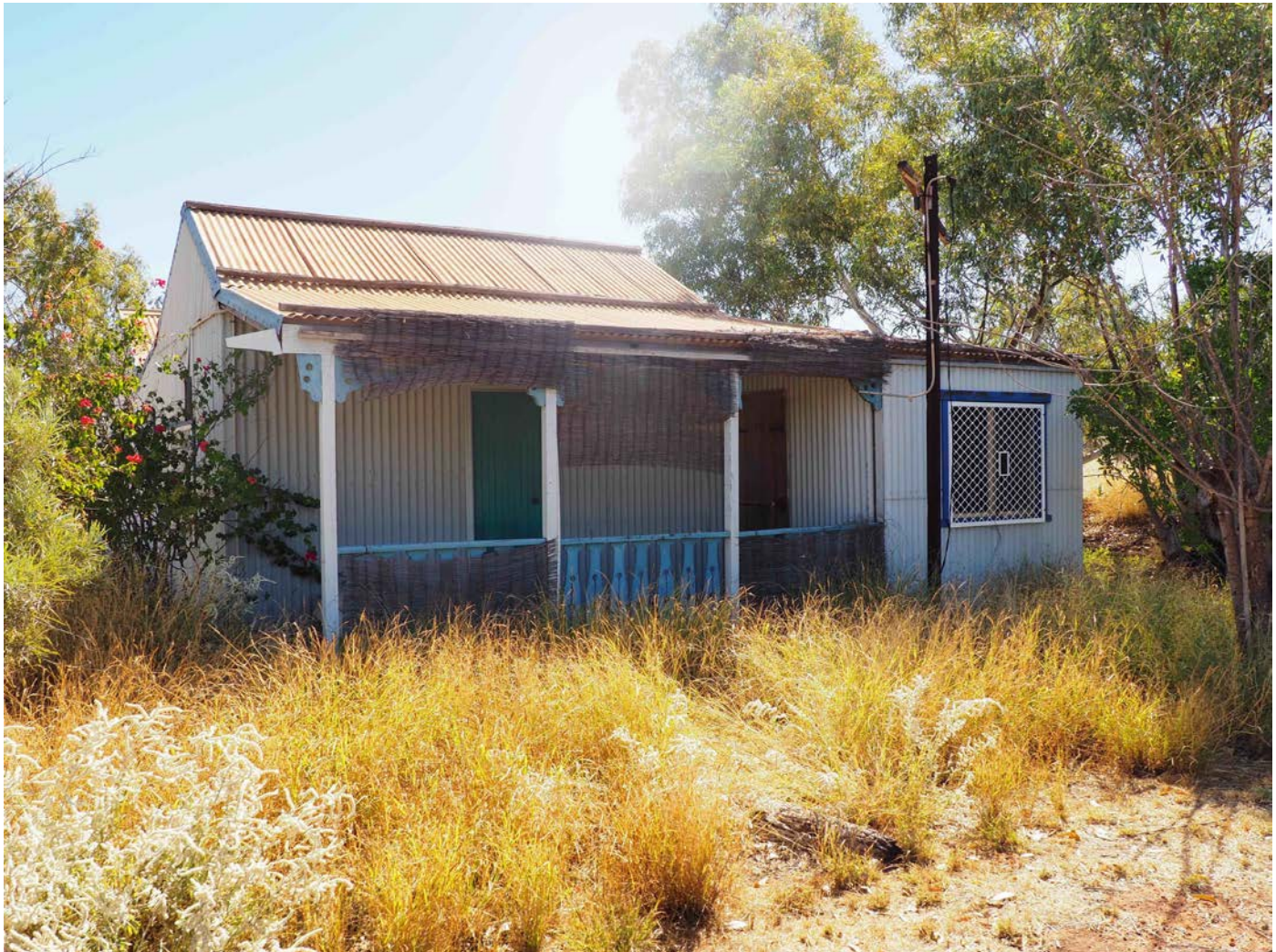
The residence at 65 Second Avenue, Onslow 2016.
