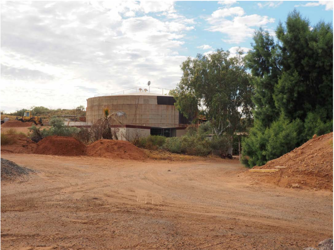
Aviation Spirit Pump Station (fmr), 2016.
