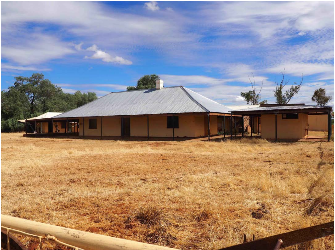
Nanutarra Homestead north wing (built c.1883/1884) 2016.
