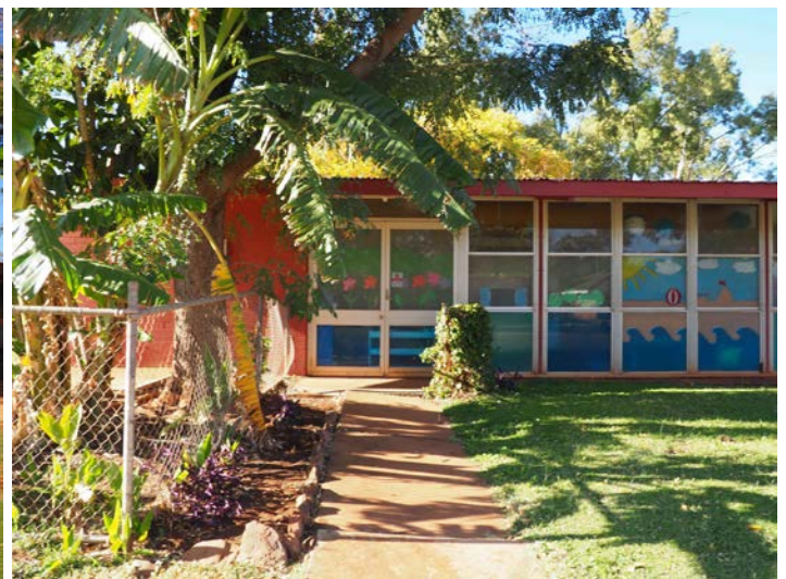
Close up of front façade, 2016.
