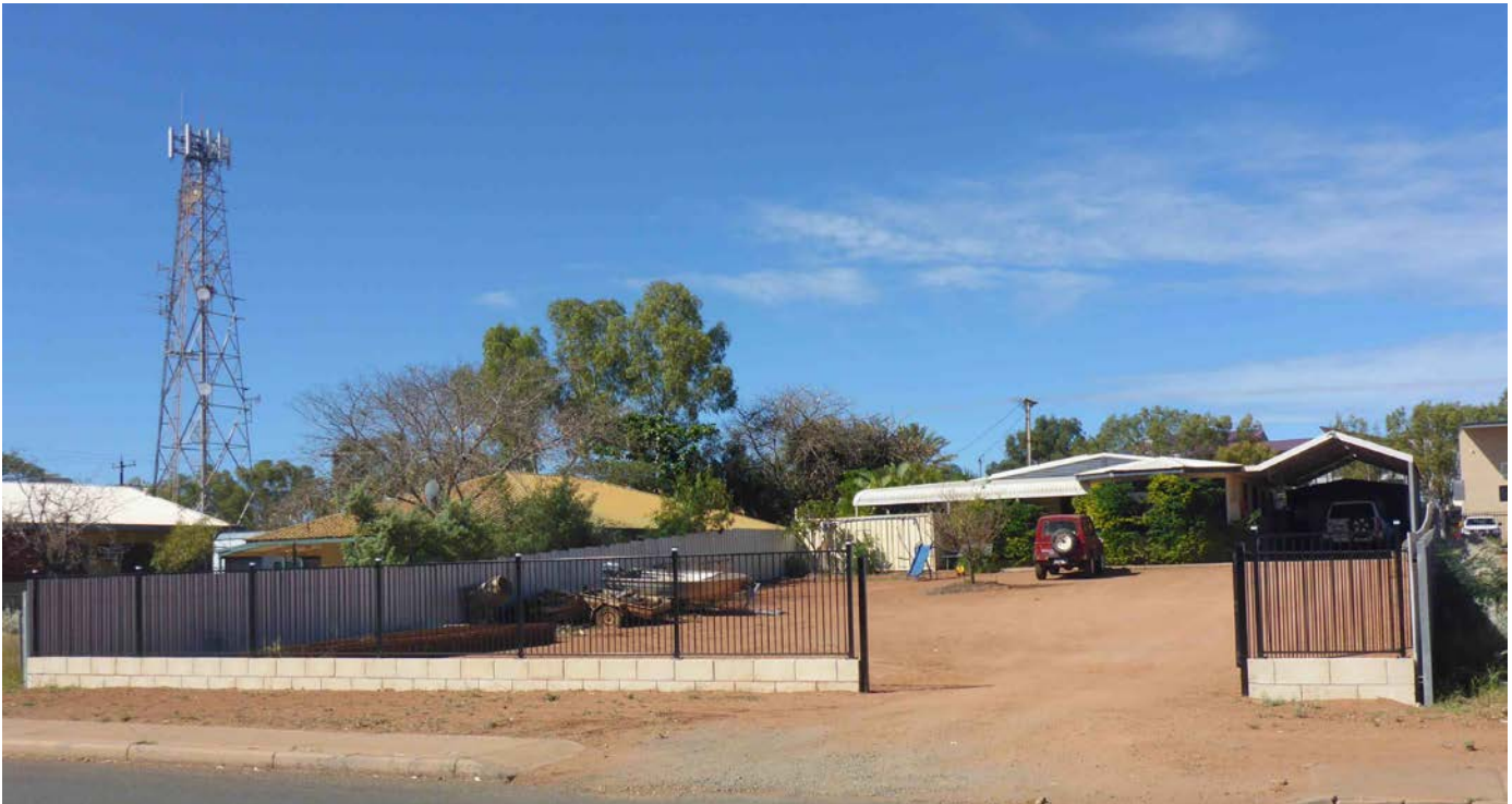
Replacement dwelling at 26 Third Avenue, Onslow 2016.
