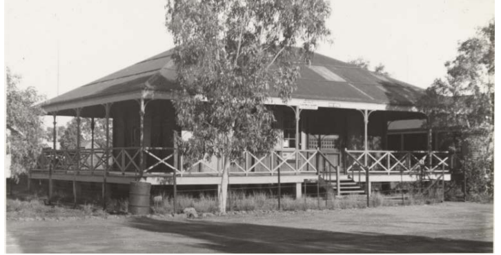
New Onslow Post Office 1939. Source: State Library of Western Australia BA1289/134
