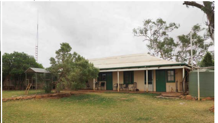
South-east corner of Homestead, 2016.
