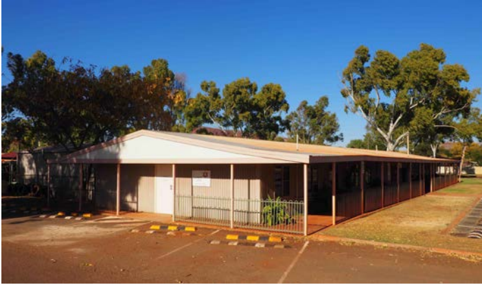
Nintirri Centre (northern building). Source: TPG October 2016
