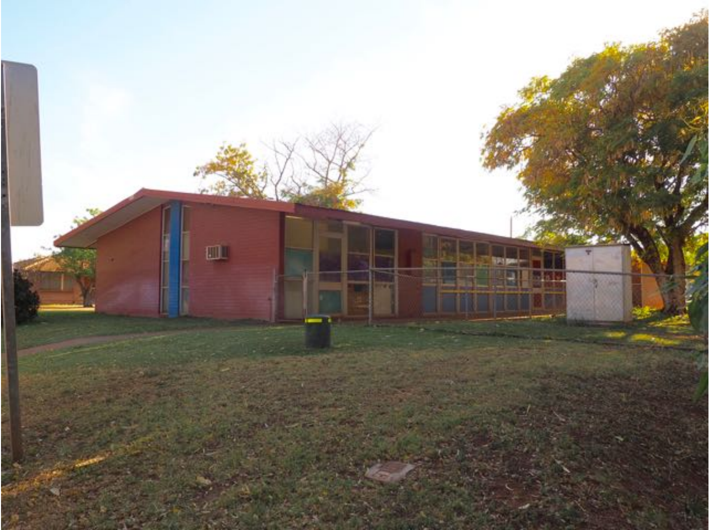
Western (side) and southern (rear) elevations, 2016.
