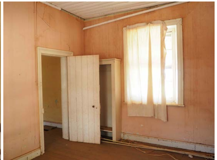
Eastern room of the north wing 2016.
