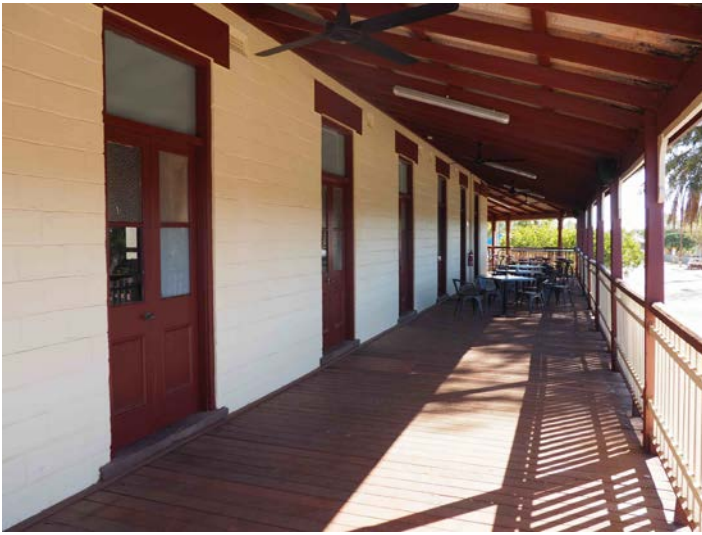
Beadon Bay Hotel first floor verandah, 2016.
