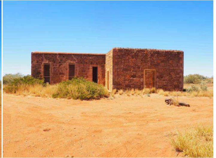
Old Onslow Gaol 2016.
