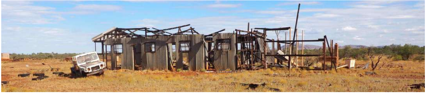
Accommodation Building/Shearers Quarters at the Shearing Camp 2016.
