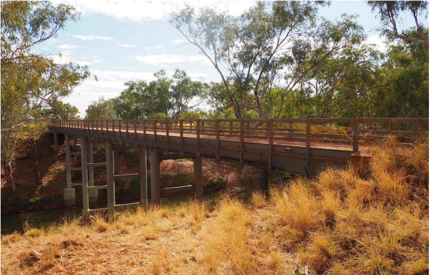
Ashburton Road River Bridge, 2016.
