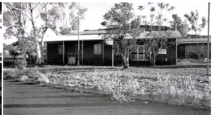
Right image: Wittenoom Police Station/Court House 1995 (built 1964, demolished 1996). Source: National Trust of Western Australia (1995)
