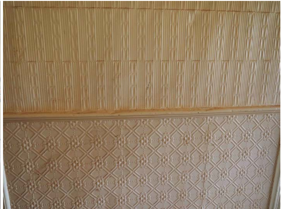
Decorative pressed tin wall cladding, 2016.
