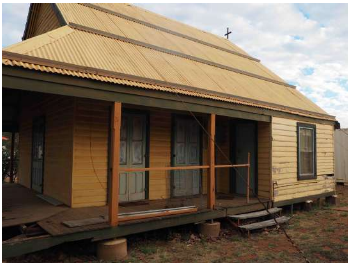
Side (north-west) elevation of church, 2016.
