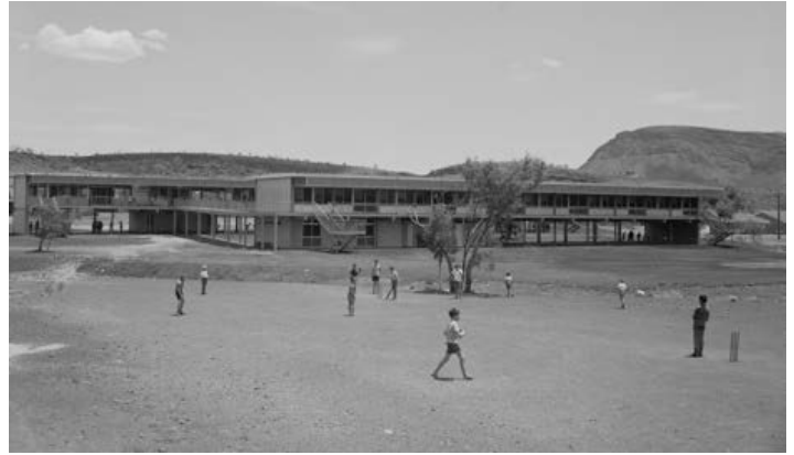
Right image: Tom Price Primary School 1966 after extension and construction of new wing. Source: State Library of Western Australia 267,284PD
