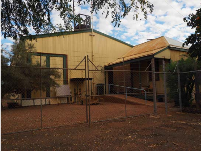
Northern end of Goods Shed showing attached office, 2016.
