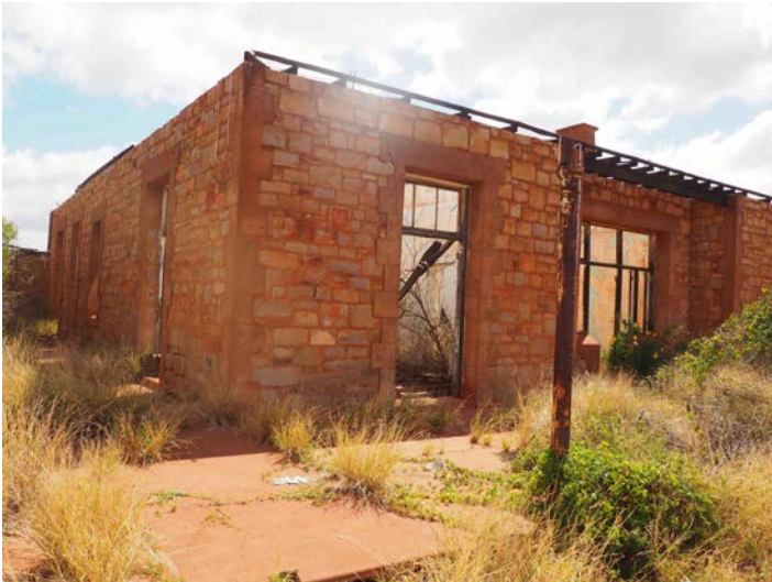
Remnant verandah post and window detailing, 2016.
