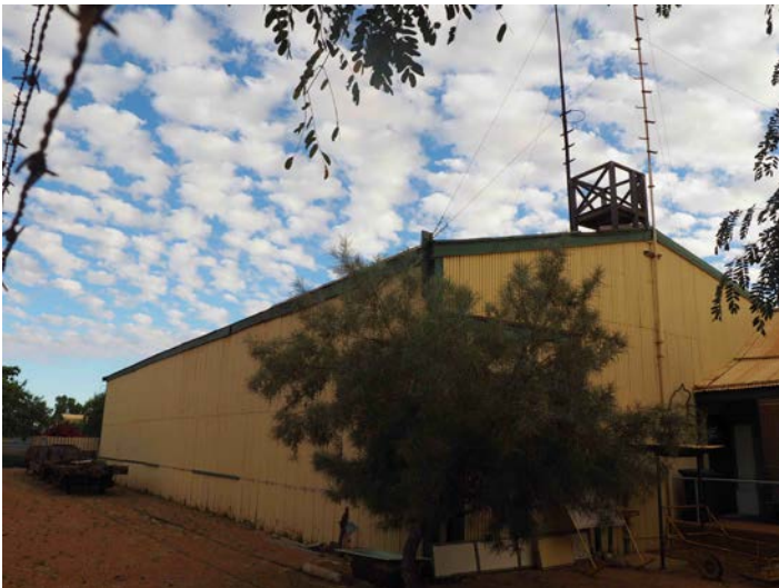
Eastern elevation of Goods Shed, 2016.
