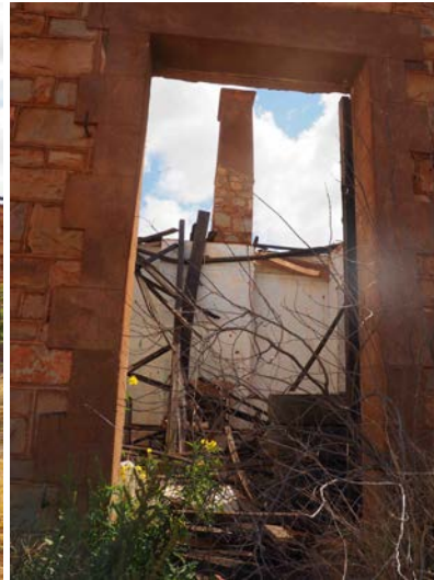
Fireplace and chimney, 2016.
