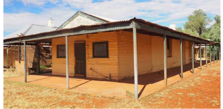
Rear and side (western) elevation of the south wing 2016.
