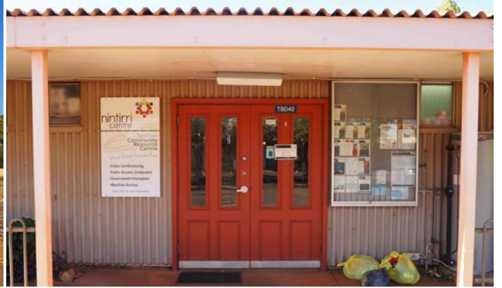
Nintirri Centre (northern building). Source: TPG October 2016
