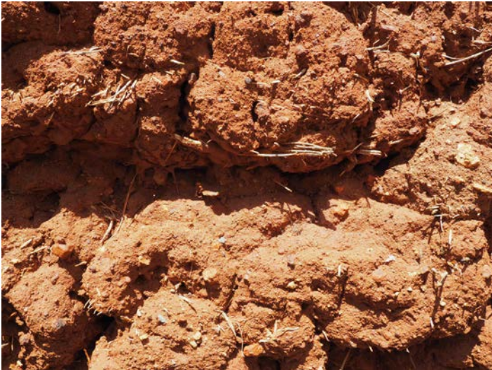
Close up of mud brick, 2016.
