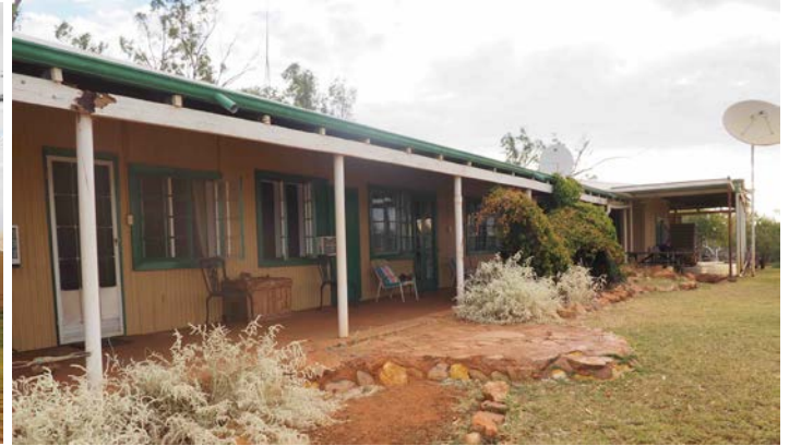
Close up of front façade of Homestead looking west, 2016.
