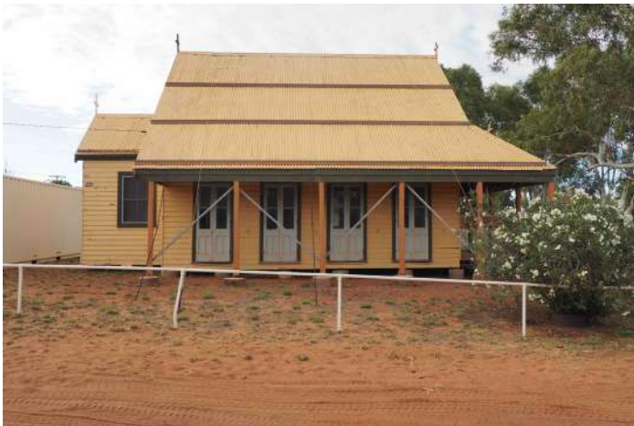
Simpson Street elevation of church, 2016.
