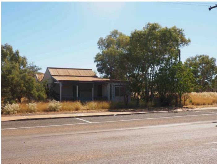
View of front elevation from Second Avenue 2016.
