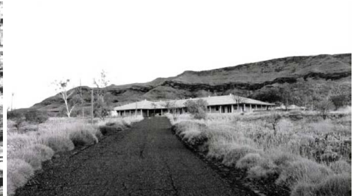
Right image: Wittenoom Hospital 1995 (built 1950, demolished 1995). Source: National Trust of Western Australia (1995)
