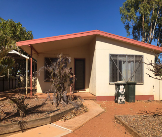
583 Third Ave Onslow (Proposed Demolition)
