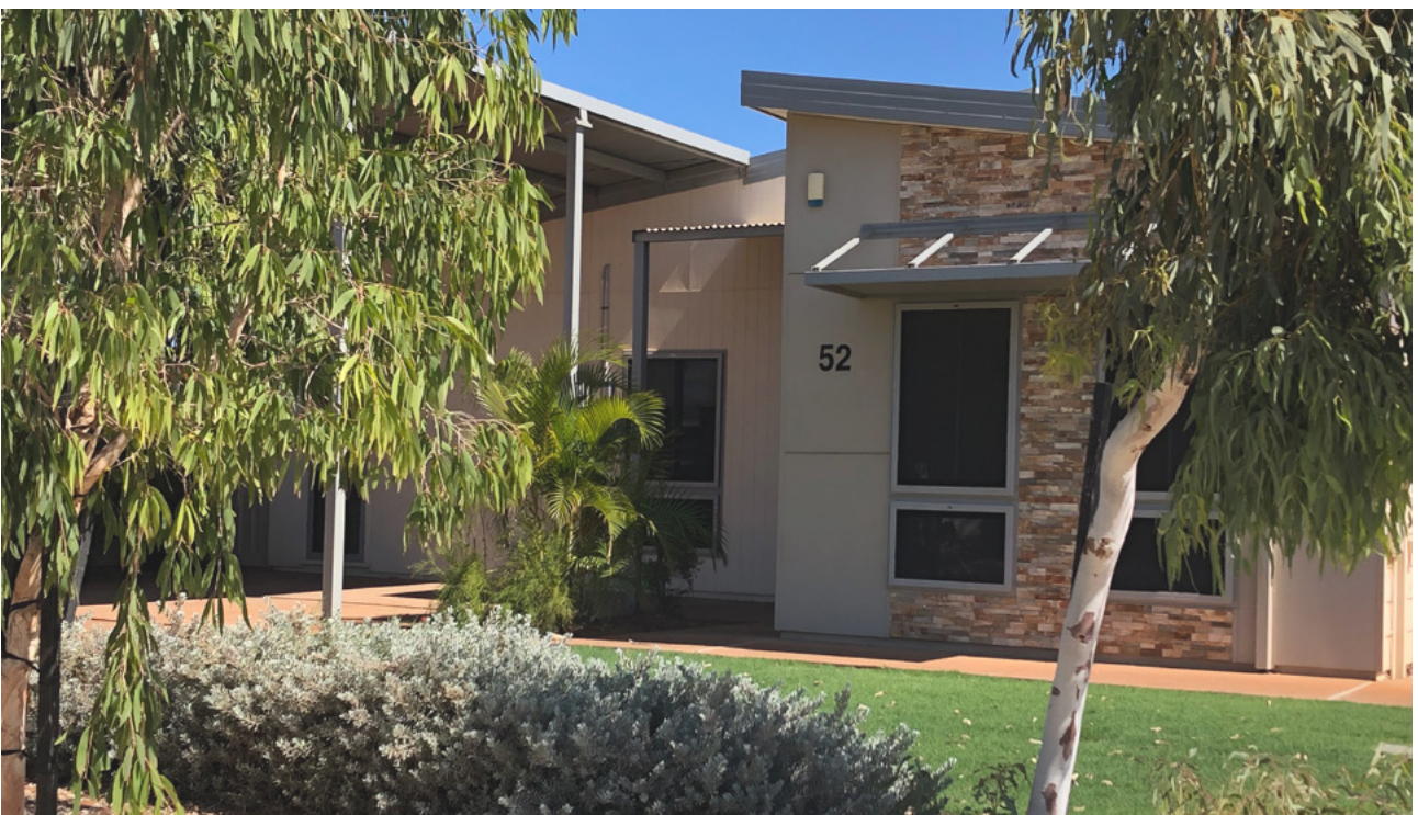
6 Carlyon, Onslow - New Build
