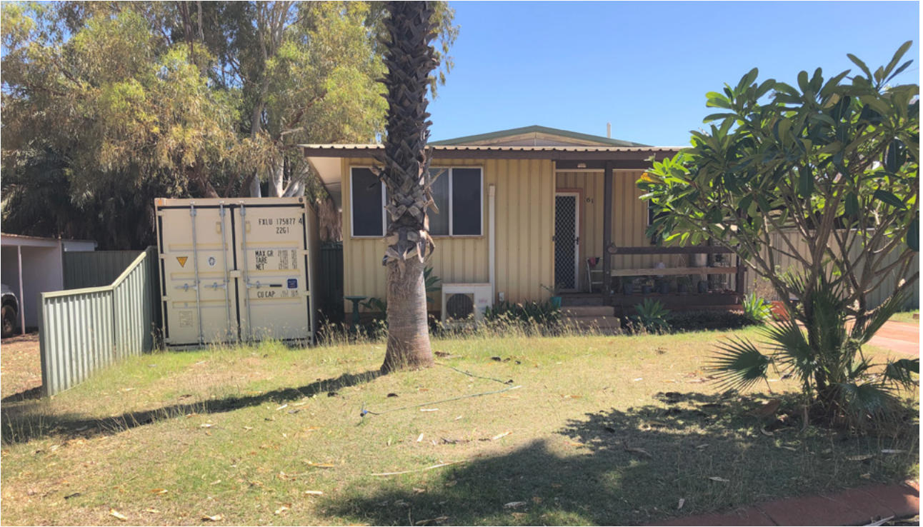
61 Pine Street, Tom Price - Potential Demolition and Rebuild
