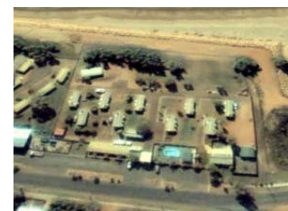
Aerial view of Sun Chalets
