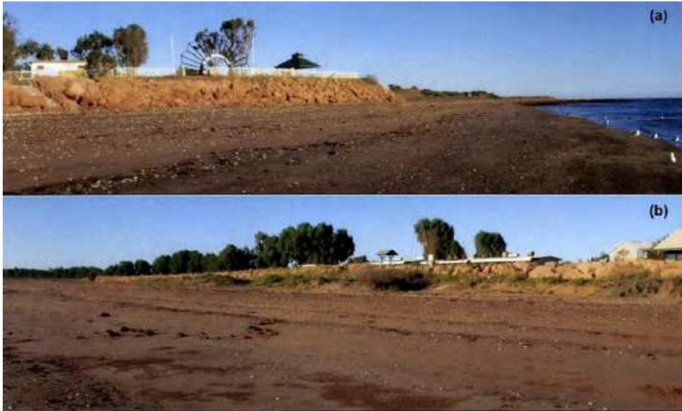
Figure 1 – Seawall Protection at the Adjacent Beach
