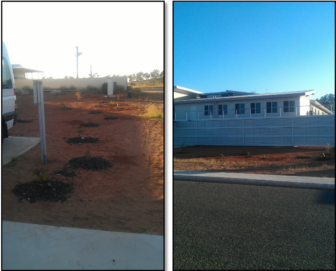
Landscaping undertaken by the developer – Photo taken 22 August 2013
