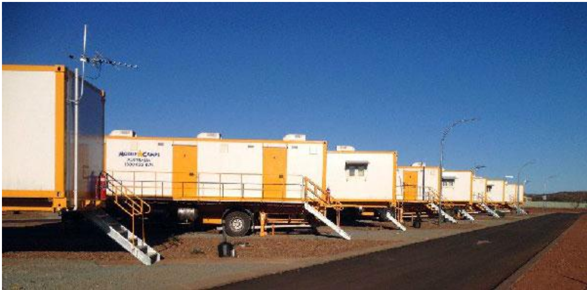
Figure 1: Existing 40 Man Village Using Mobile Accommodation Units at Paraburdoo for Rio Tinto.
