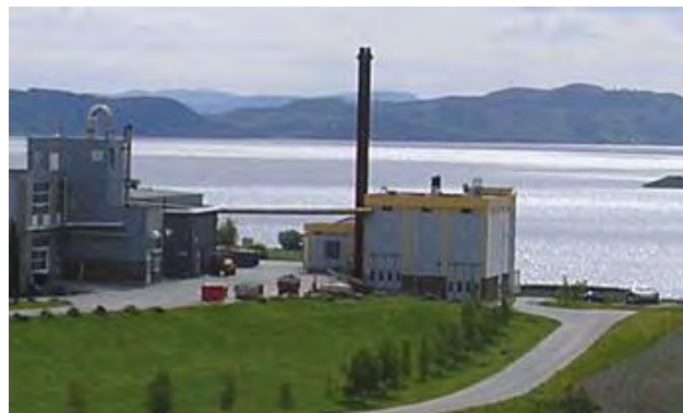
Plate 10-7: OE Gasification plant in Norway
