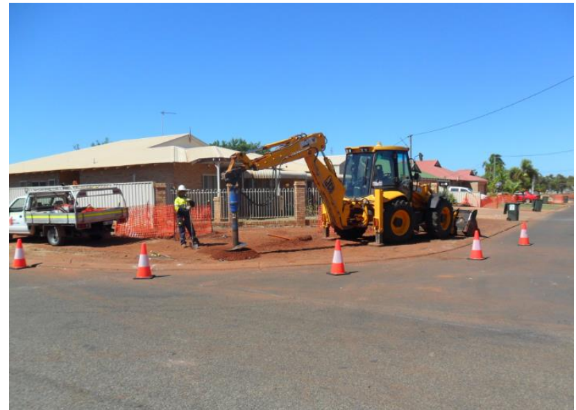
Hole boring for streetlight installation
