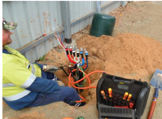
Cables being prepared for energisation
