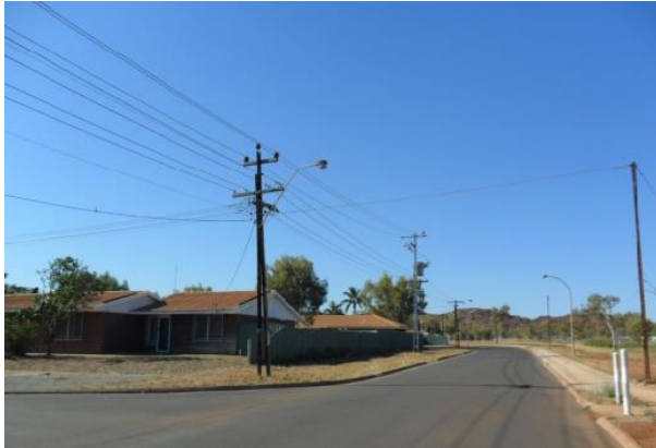
Before underground power
