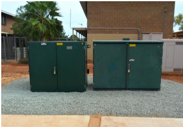
Transformer installation
