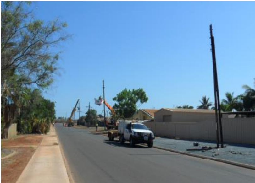
Removal of overhead powerlines
