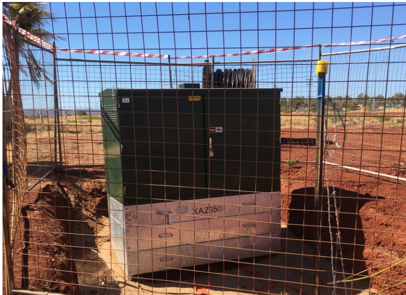
Transformer installation
