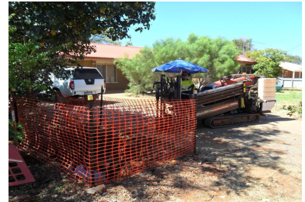
Directional drilling for consumer conduit installation
