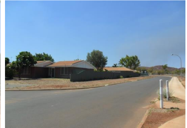
Underground power works complete
