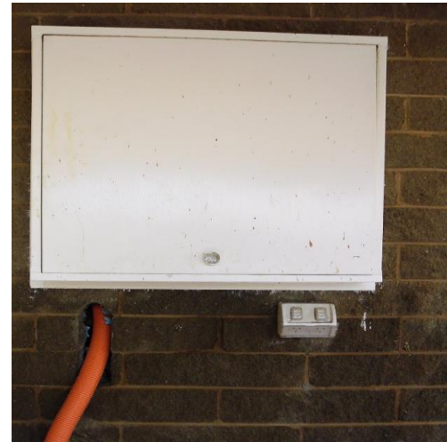
An entry point for the cable is made in the wall under the meter box
