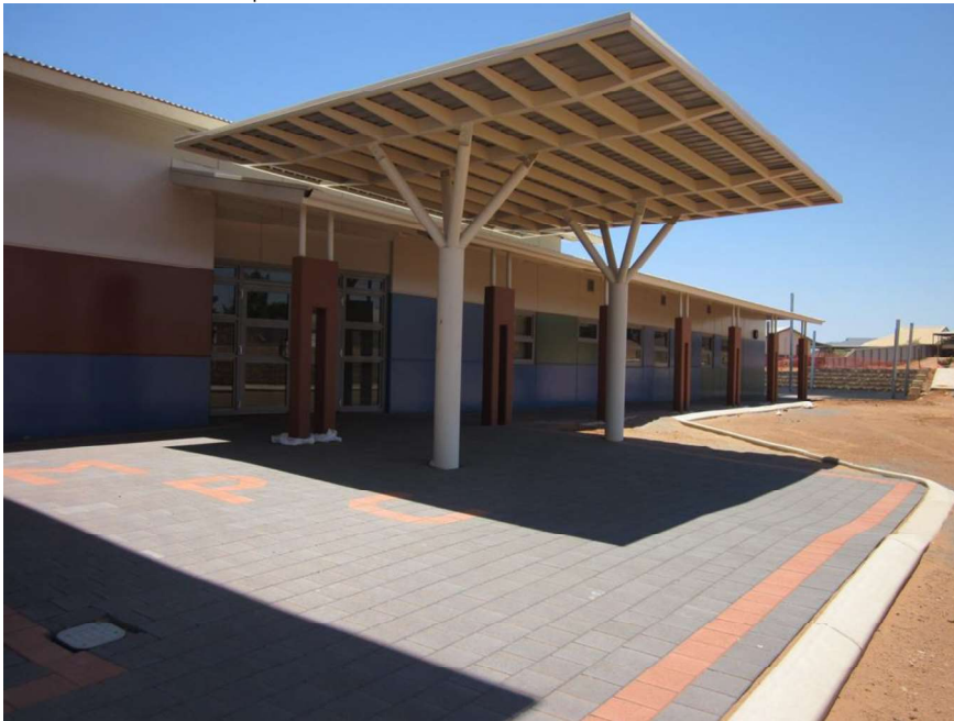
Onslow Multi-Purpose Centre
