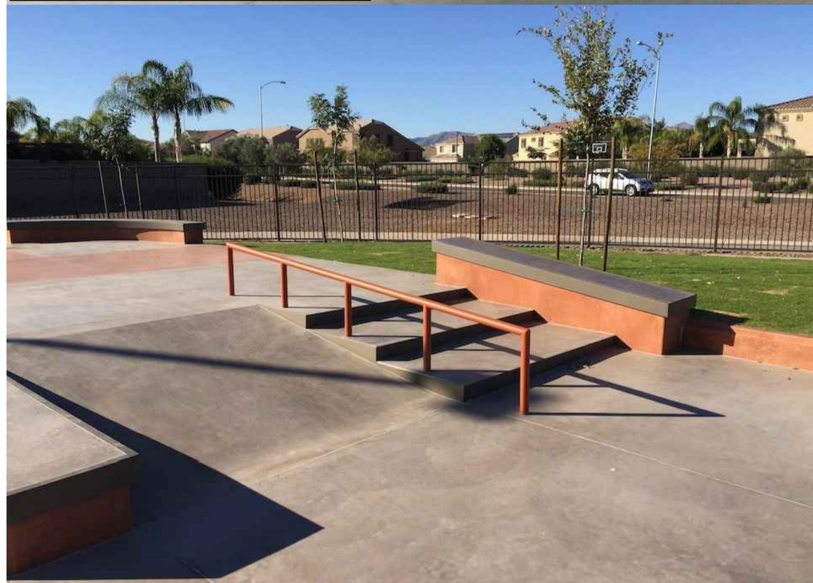
COMBINATION STREET STYLE BANK AND STAIR SET WITH DOWN RAIL AND LEDGE
