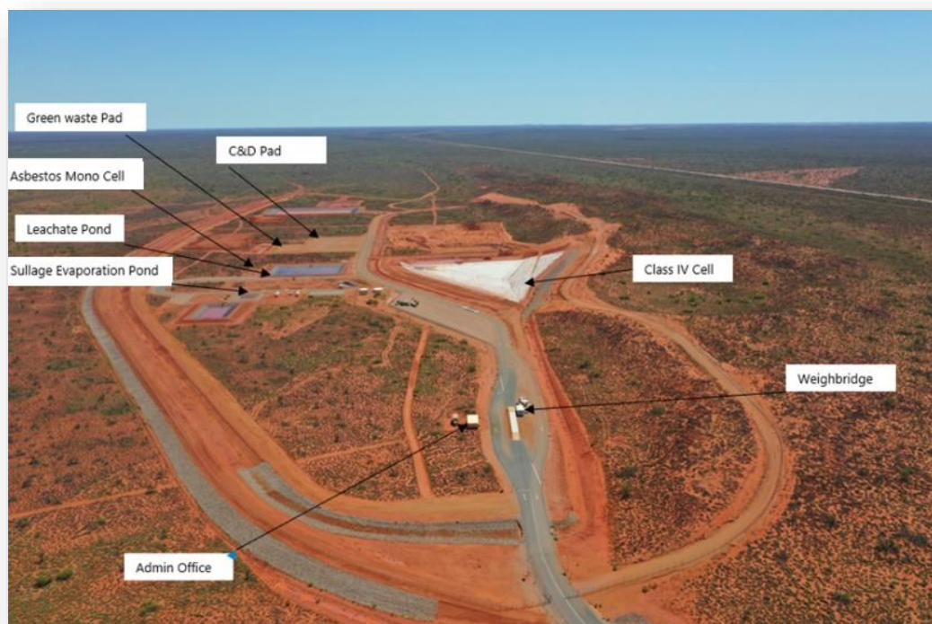
Figure: Onslow waste transfer station – Class-IV.
