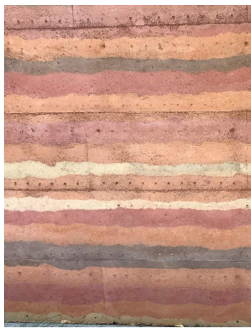
RAMMED EARTH FEATURE MATERIAL
