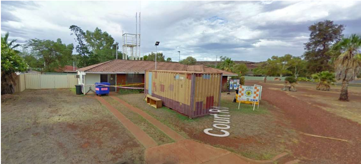
Figure 2 Existing Building Street Elevation (Google Street Maps Extract)
