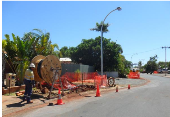
Mains cable installation
