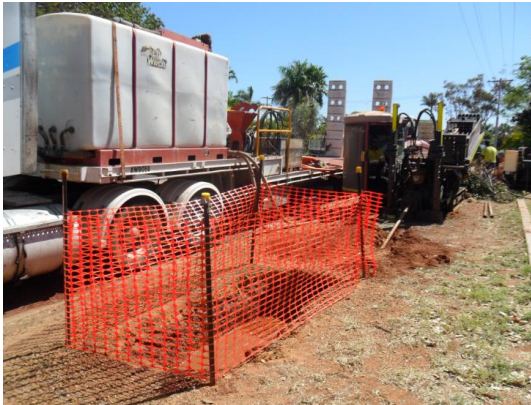
Directional drilling for mains conduit installation
