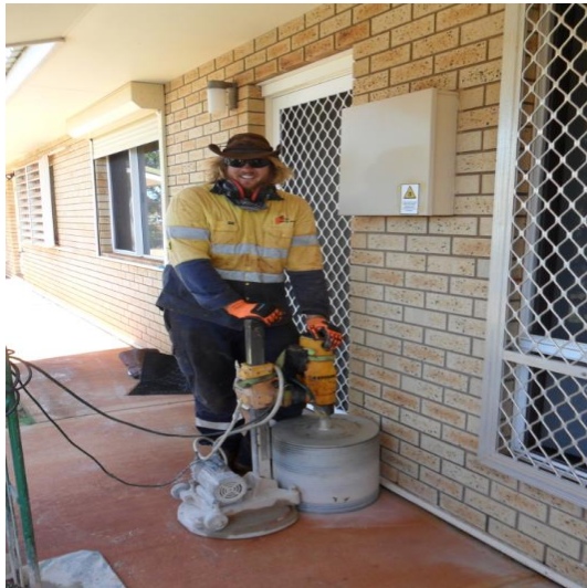
Core boring used for concrete cut out
