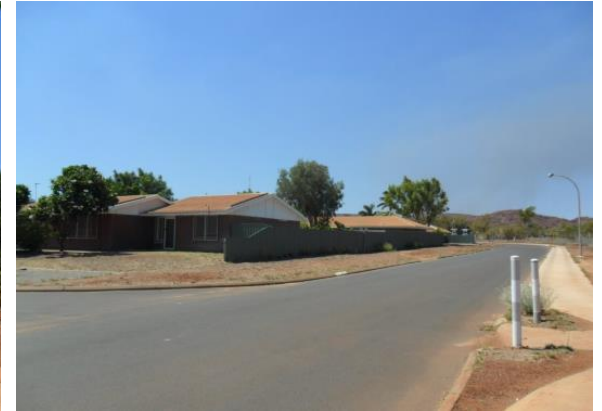
Underground power works complete
