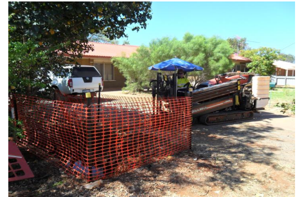
Directional drilling for consumer conduit installation
