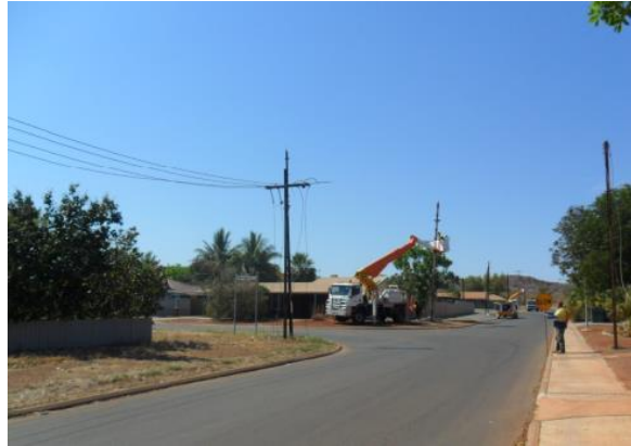
Removal of old powerlines
