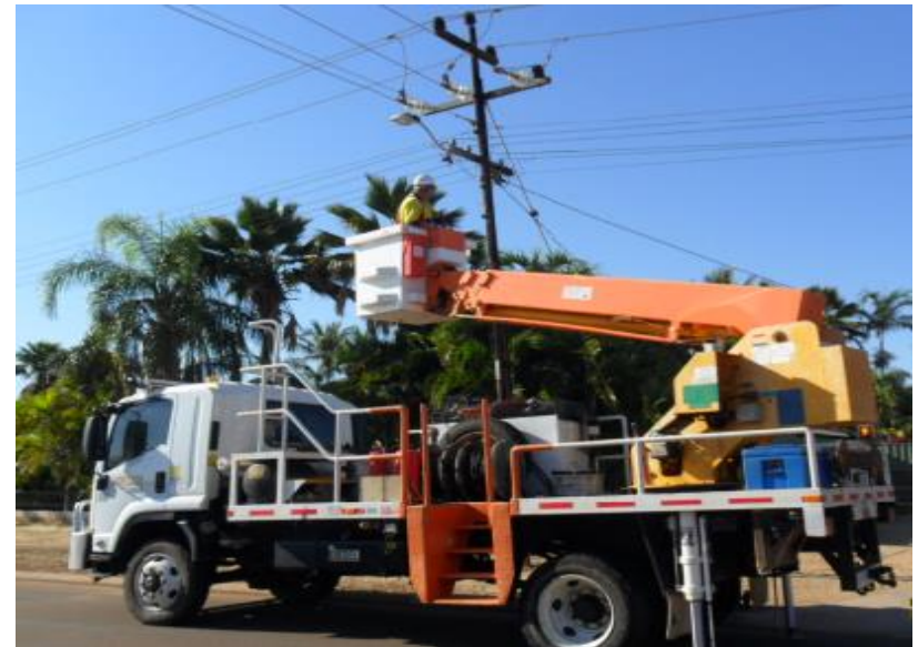
Removal of overhead powerlines
