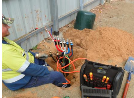
Cables being prepared for energisation
