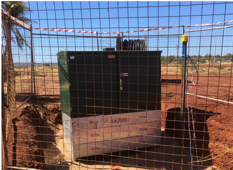
Transformer installation
