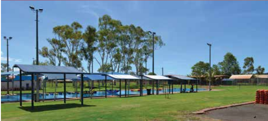
Shade structures at Paraburdoo swimming pool
