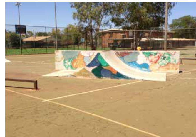
Prefabricated Steel Features - CONVIC site photos
