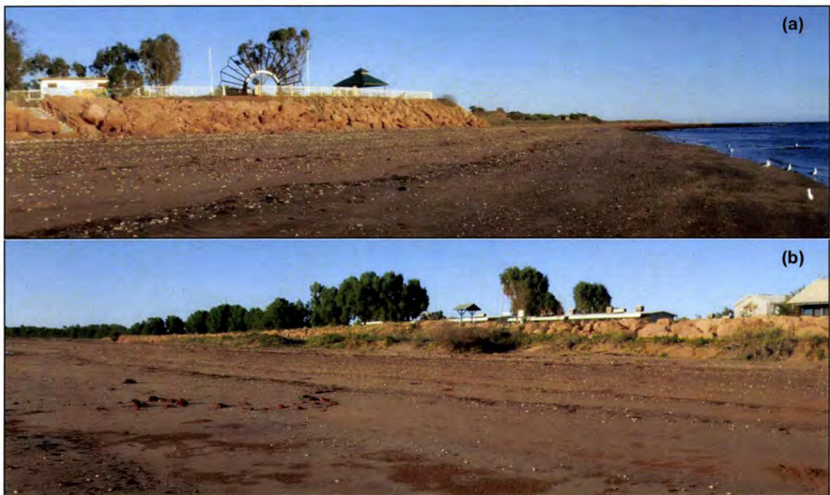
Figure 1.6 - (a) Western end of Seawall, (b) Eastern end of Seawall
