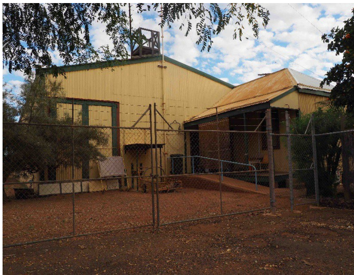
Northern end of Goods Shed showing attached office, 2016.
