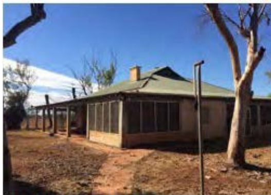
Homestead infilled verandah, 2017
