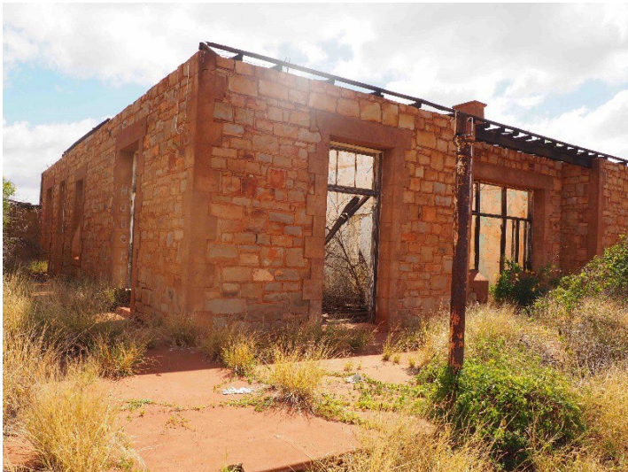
Remnant verandah post and window detailing, 2016.
