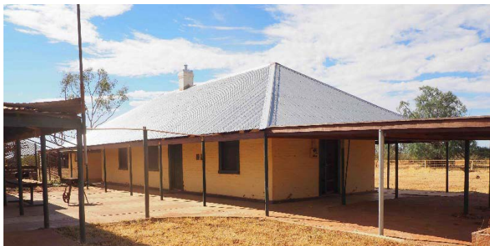
Rear elevation of the north wing 2016.
