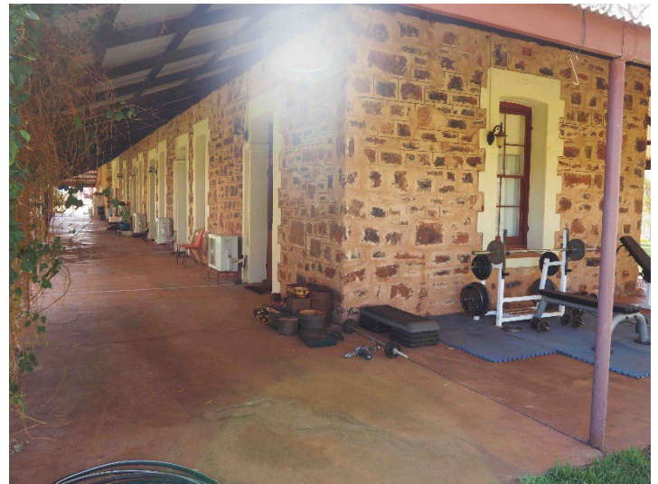
Hamersley Homestead side and rear elevations, 2016.
