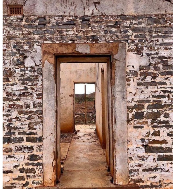
Figure 4 – Existing condition of the interior and doors
