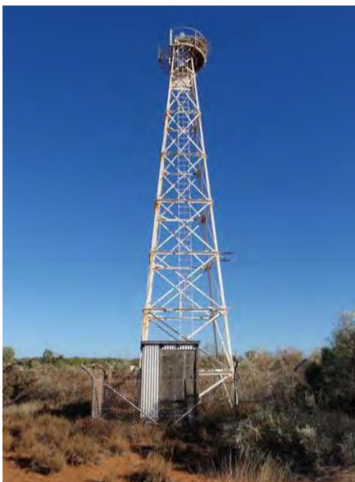
Photo. Beadon Creek Rear Lead Tower – View from south showing all nine sections, supply shed on south side and protective fencing around base. (2012). Source: Menck, Archival Record , 2019.
