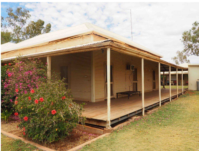
Western elevation of Yanrey Homestead, 2016.
