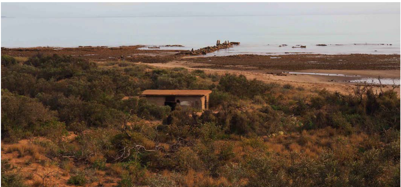
Pump Out Station and remains of Onslow jetty beyond, 2016.
