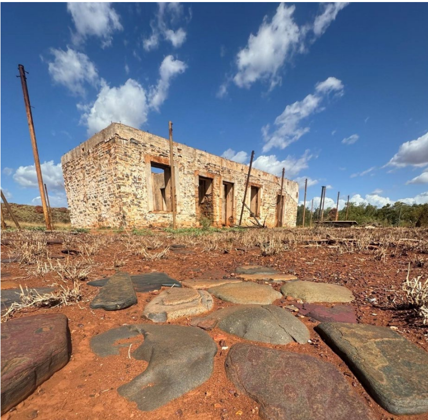
Figure 2 – West elevation of the Deepdale Homestead.
