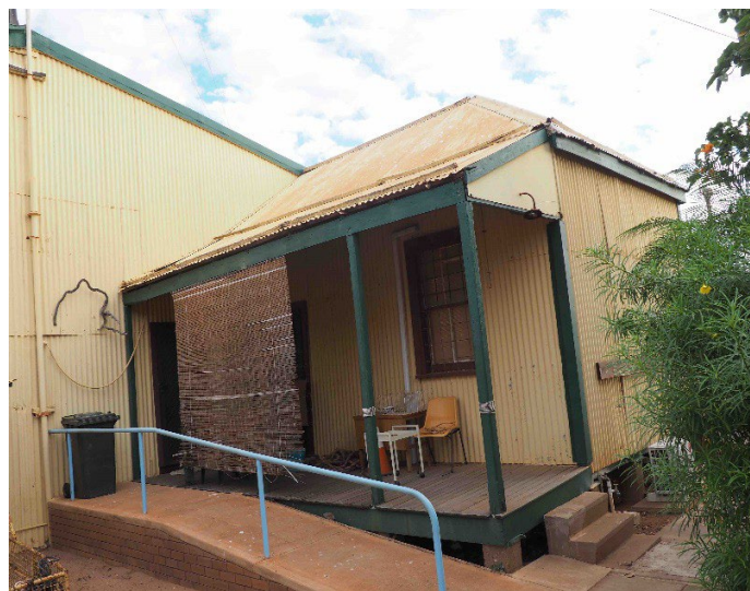
Close up of office, 2016.
