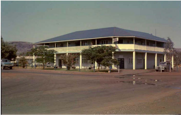
Left Image: Fortescue Hotel, Wittenoom, 1966 (built 1947, demolished 1996). Source: State Library of WA
