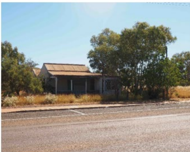
View of front elevation from Second Avenue 2016.
