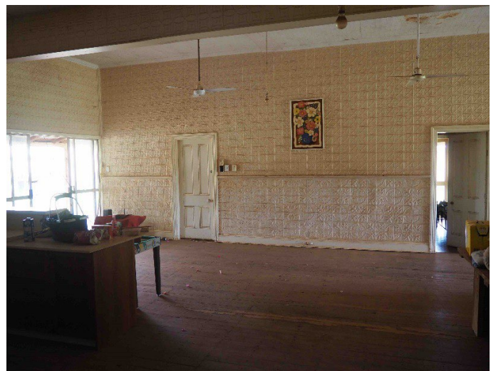
Central internal living space, 2016.
