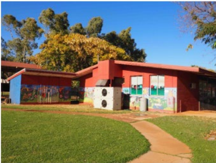
Eastern (side) elevations 2016.
