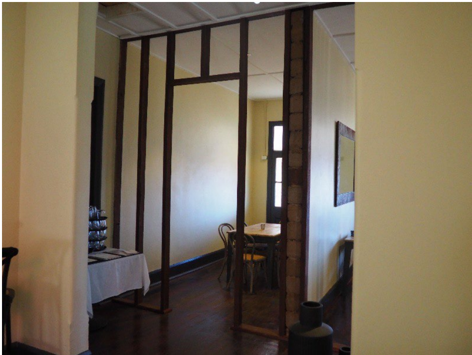
Interpretation of former bedroom through retention of timber frame, 2016.
