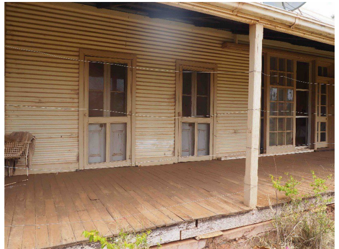
Close up of front elevation of Yanrey Homestead, 2016.
