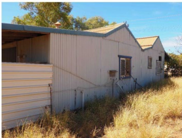
View of side (eastern) elevation from Second Avenue 2016.
