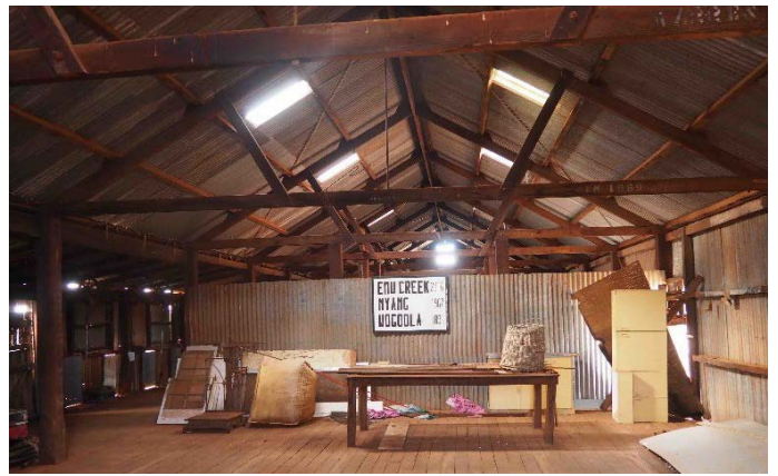
Inside view of Shearing Shed, 2016.
