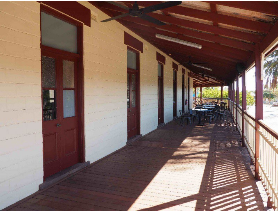
Beadon Bay Hotel first floor verandah, 2016.
