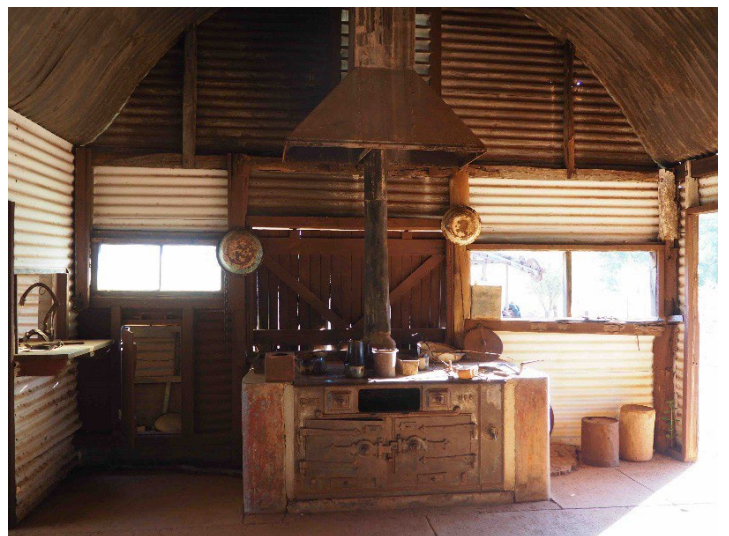
Internal view of kitchen, 2016.
