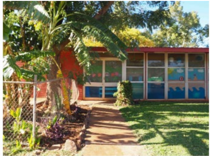
Close up of front façade, 2016.
