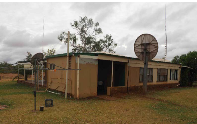
South-west corner of Homestead, 2016.
