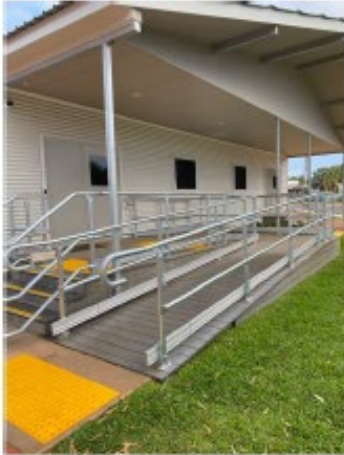
Disability ramp access
