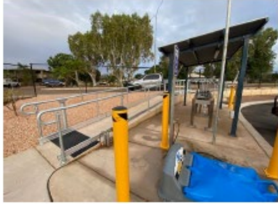
Fish Cleaning Station Ramp
