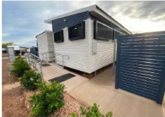
Ablution ramp, rail and pathway
