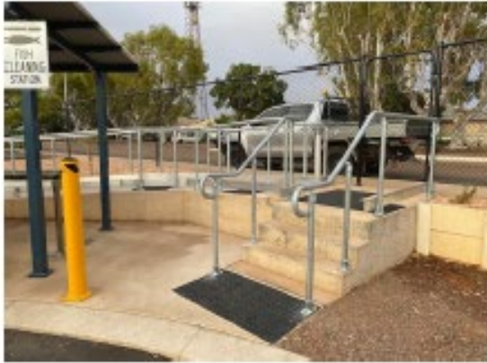
Fish Cleaning Station Ramp
